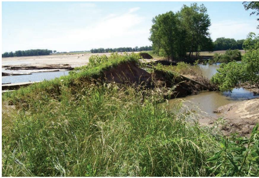
and underlying outwash parent material to depths of 3 to 6 m (10 to 20 ft) below the base of the earthen levee when the levees broke (figure 5). The force of the rushing water uprooted trees growing between the river and the levee prior to the break and deposited them on the previously protected floodplain (figure 6). The 2008 crop on the floodplain soils behind the broken levees was a total loss.
